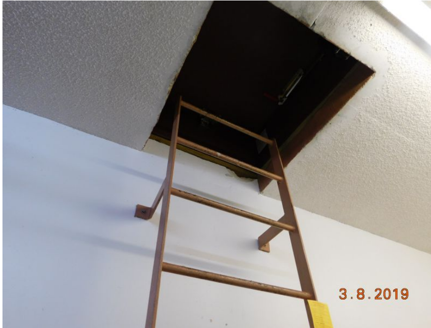
Reinforced Concrete Roof Deck
