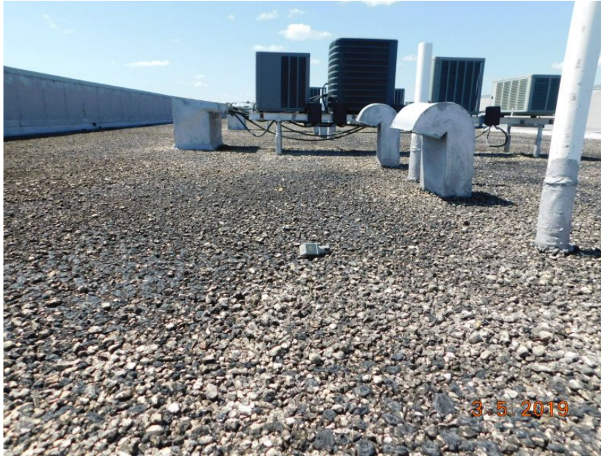
Built-Up Tar & Gravel Roof Covering
