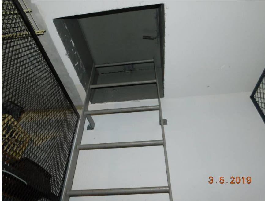
Reinforced Concrete Roof Deck
