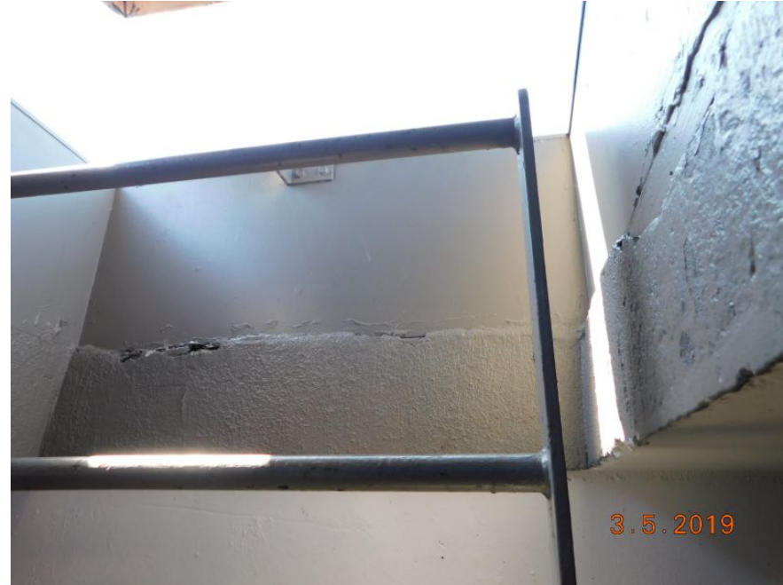
Reinforced Concrete Roof Deck
