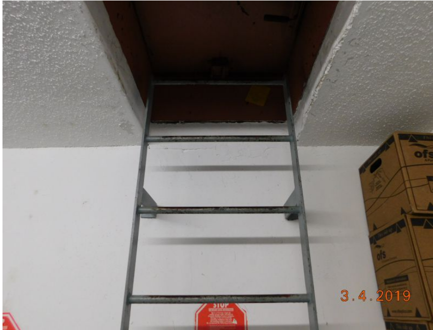
Reinforced Concrete Roof Deck
