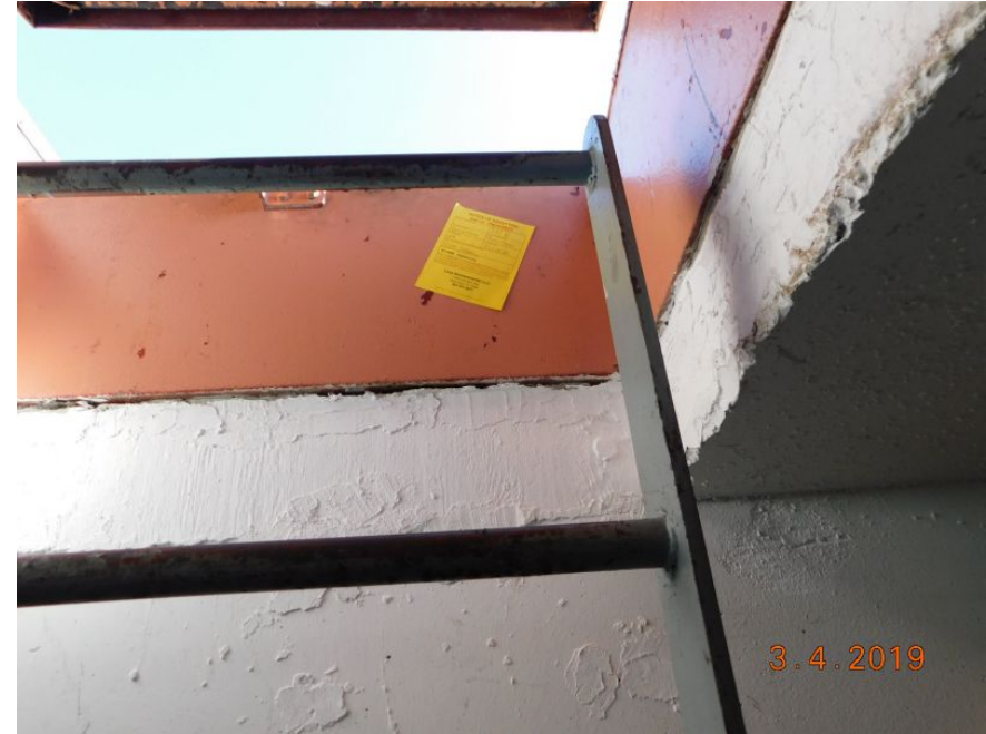
Reinforced Concrete Roof Deck
