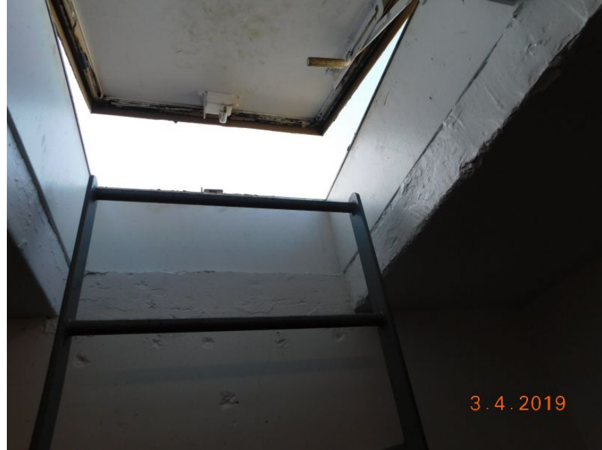
Structural Reinforced Concrete
