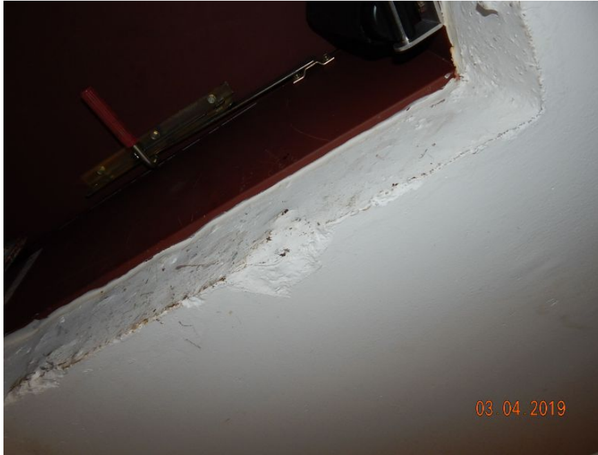
Reinforced Concrete Roof Deck
