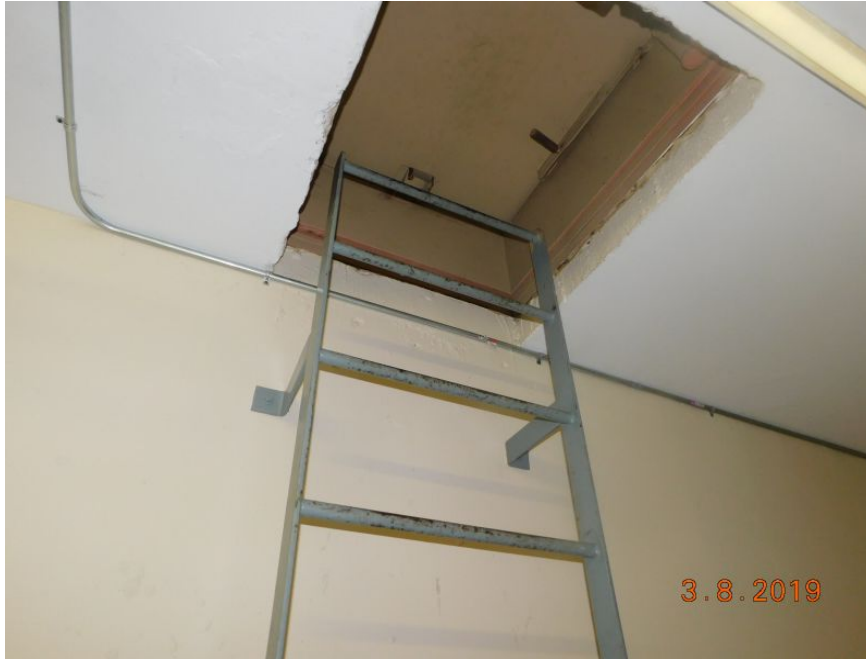
Reinforced Concrete Roof Deck
