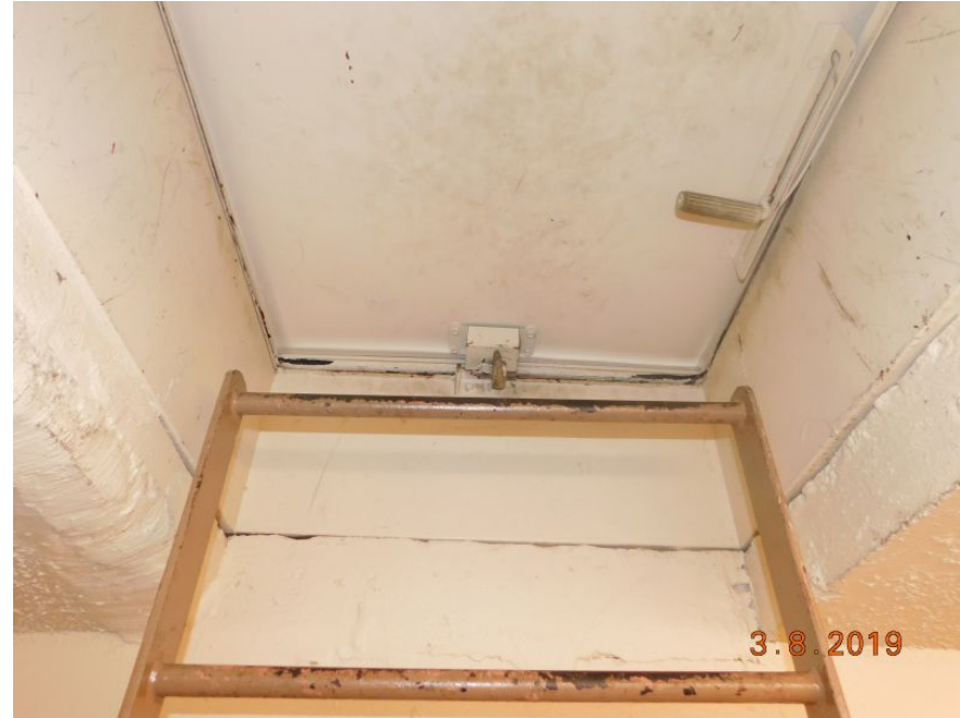
Structural Reinforced Concrete
