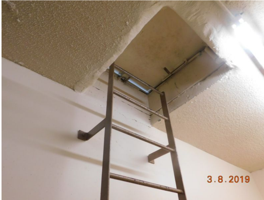
Reinforced Concrete Roof Deck
