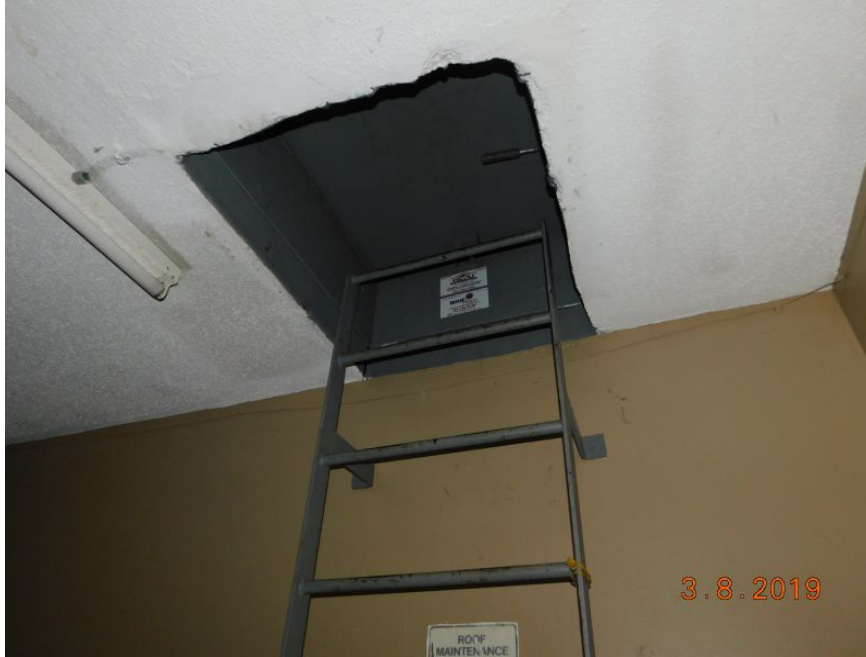
Reinforced Concrete Roof Deck
