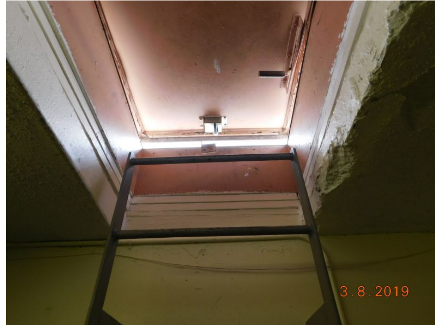
Structural Reinforced Concrete
