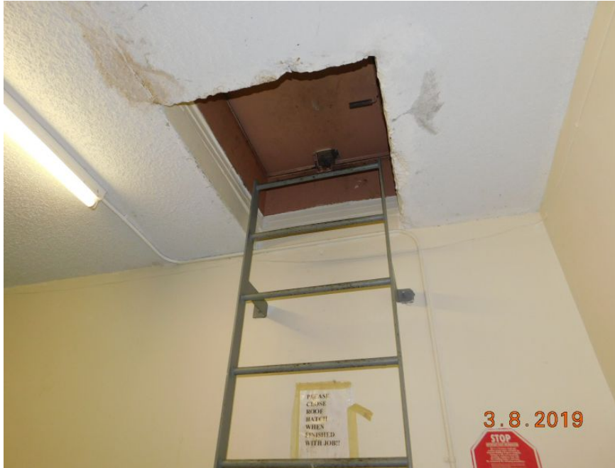
Reinforced Concrete Roof Deck
