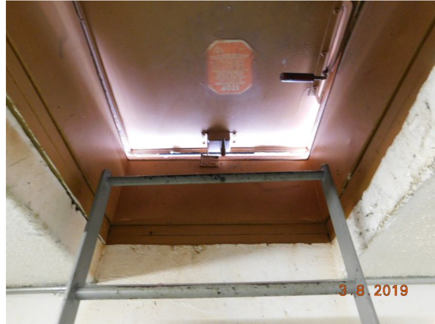
Structural Reinforced Concrete
