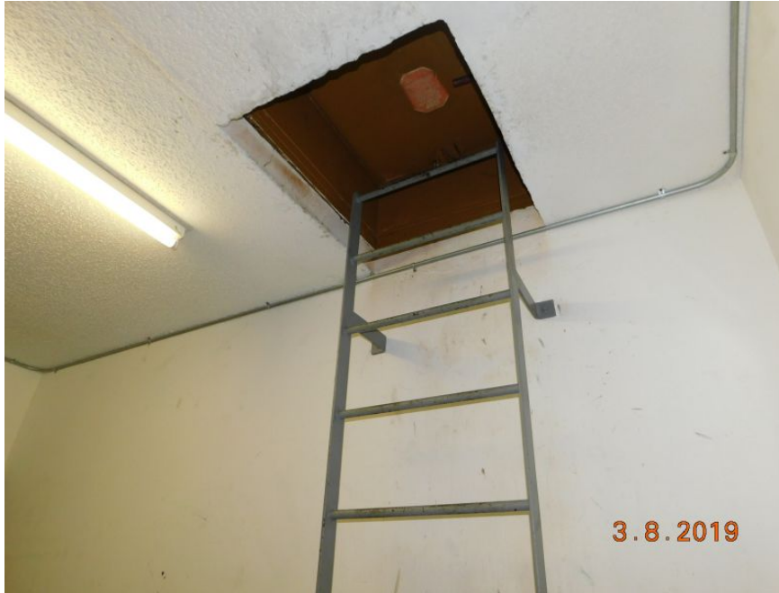
Reinforced Concrete Roof Deck
