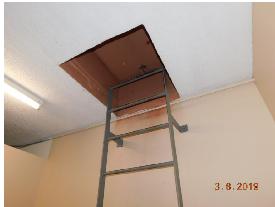
Reinforced Concrete Roof Deck
