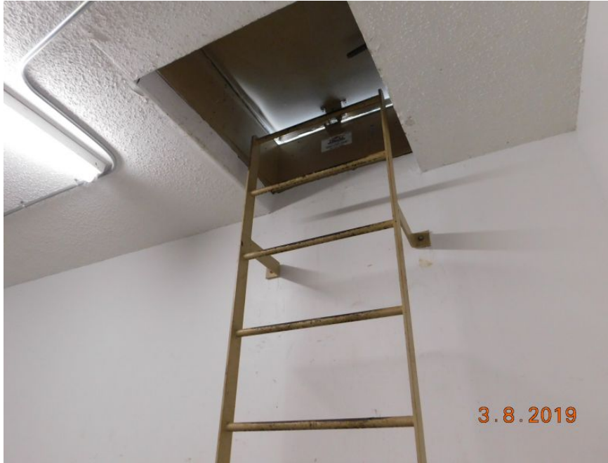
Reinforced Concrete Roof Deck
