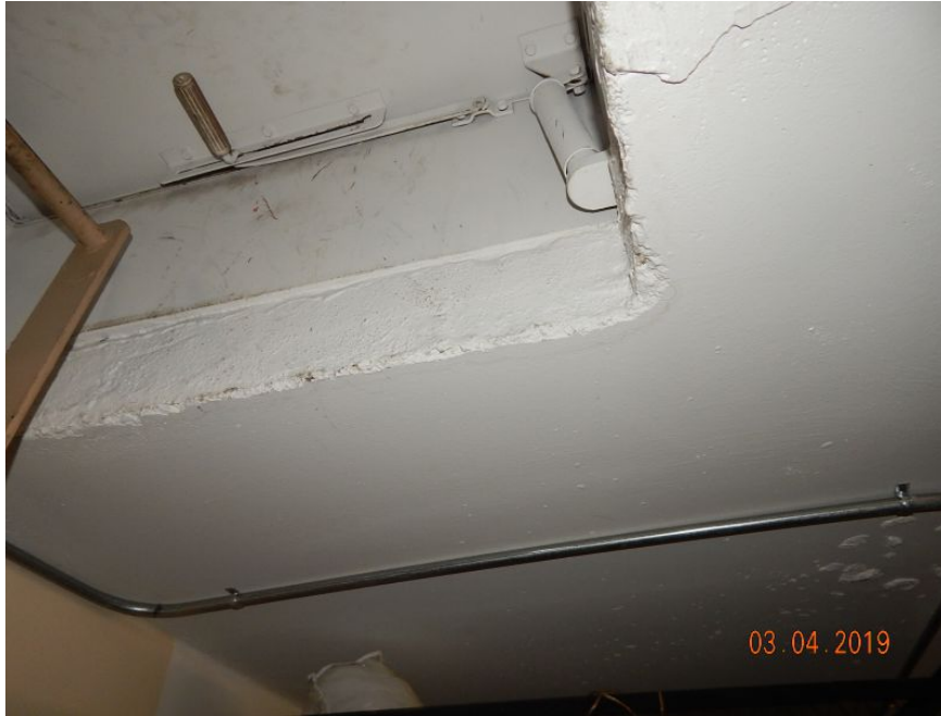
Reinforced Concrete Roof Deck
