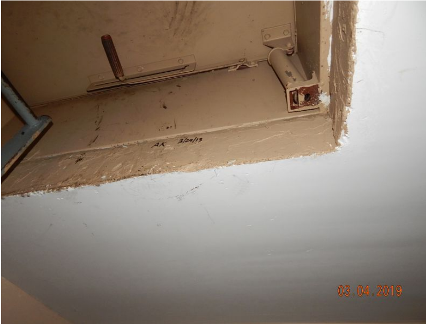
Reinforced Concrete Roof Deck
