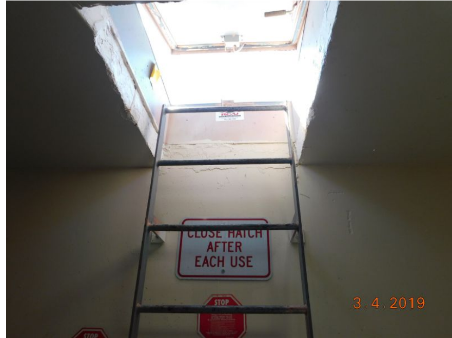
Structural Reinforced Concrete
