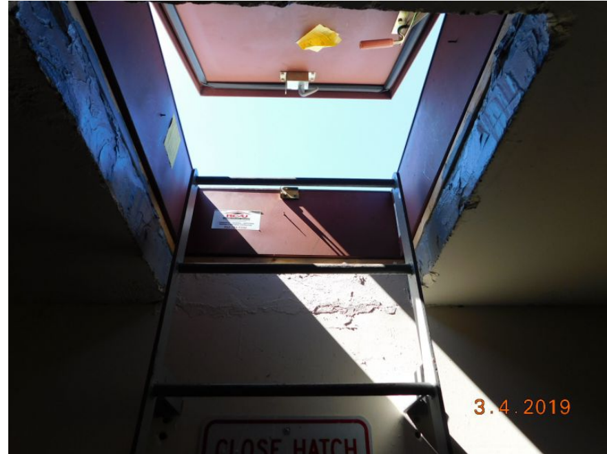
Reinforced Concrete Roof Deck
