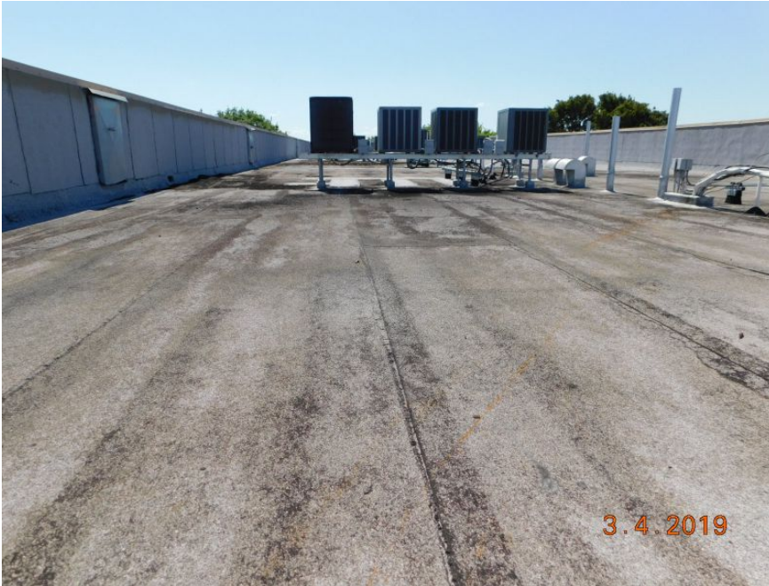
Built-up/rolled Asphalt (flat)
