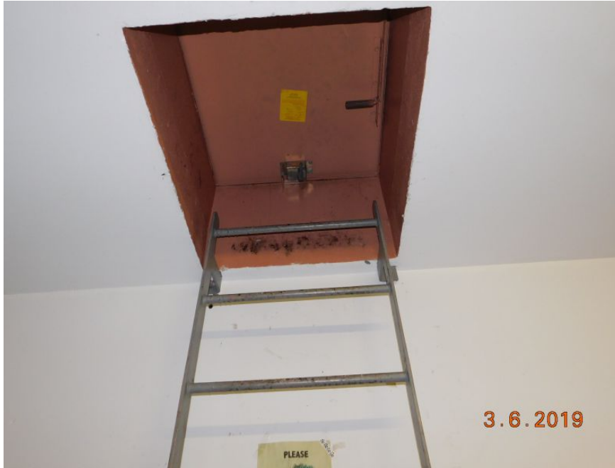
Reinforced Concrete Roof Deck
