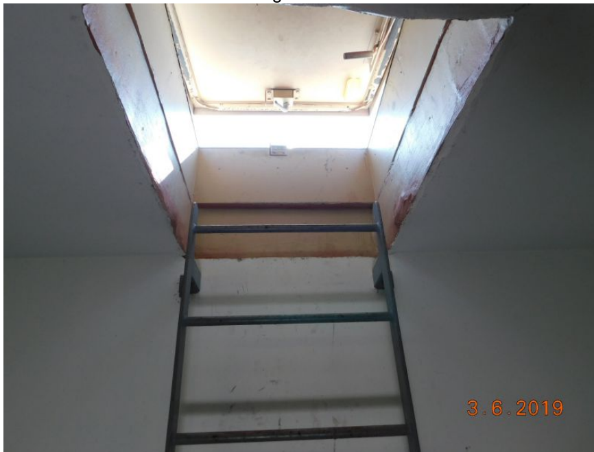
Structural Reinforced Concrete
